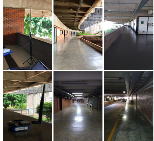
Fig. 4. Base Station, end node and floors of ICC
