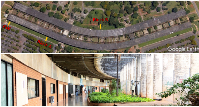
Fig. 1. Images of the Central Institute of Sciences of the University of Brasília
