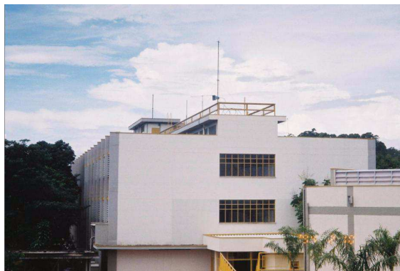
Fig. 1. Building 'E' – Faculty of Electrical and Computing Engineering. Transmitter on the rooftop.
