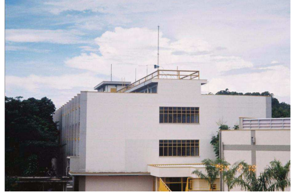
Fig. 1. Building 'E' – Faculty of Electrical and Computing Engineering. Transmitter on the rooftop.
